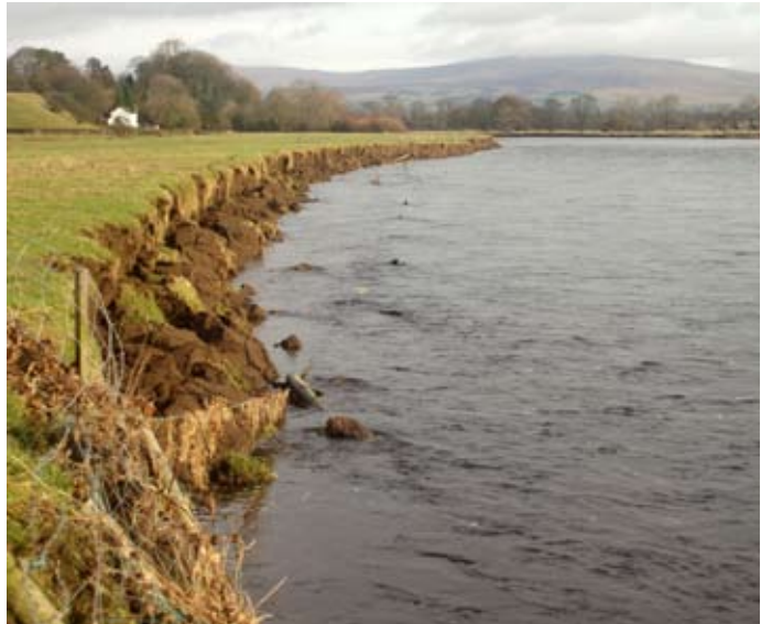
Erosion of the Lune bank near Arkholme
